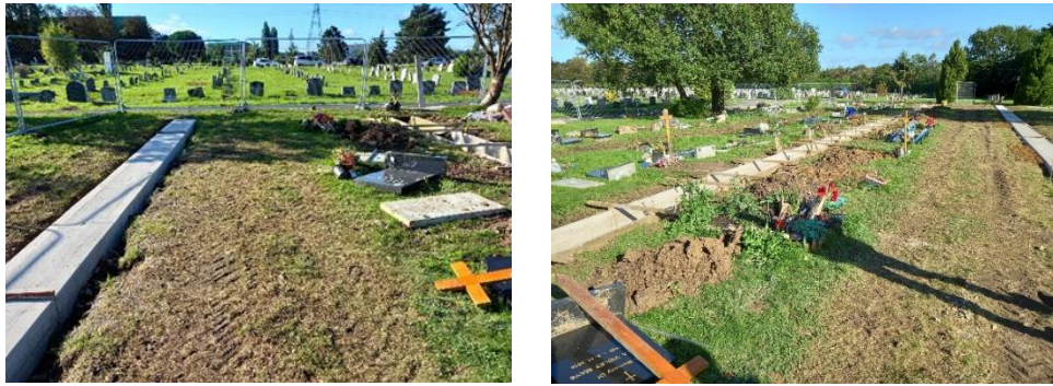
Pictures: Section F Beam Installations in progress
